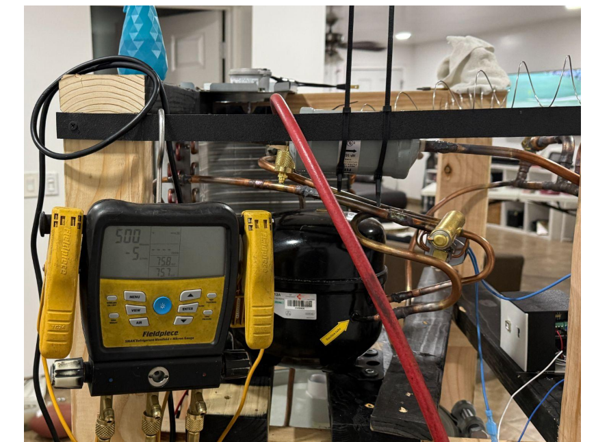
Vacuum testing to ensure system has no leaks
